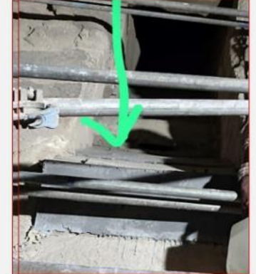
After Extension of AFR Feed Chute by 250mm Casting inside PC
