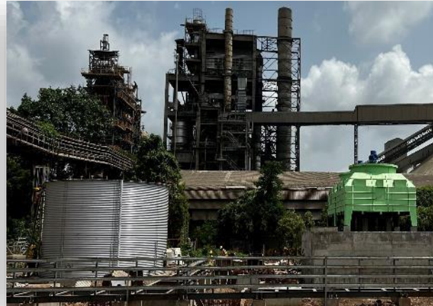
DM Tank and Auxiliary Cooling Tower
